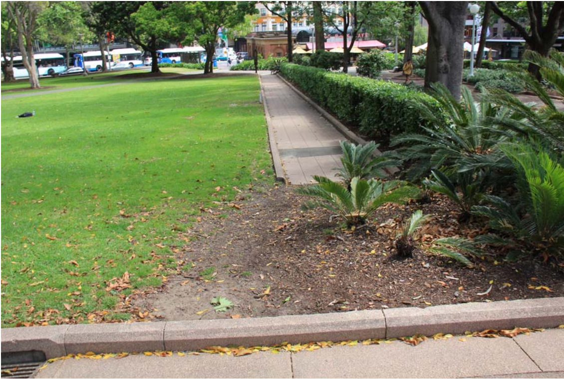
Image a) Poor accessibility - paths terminating at planting beds
