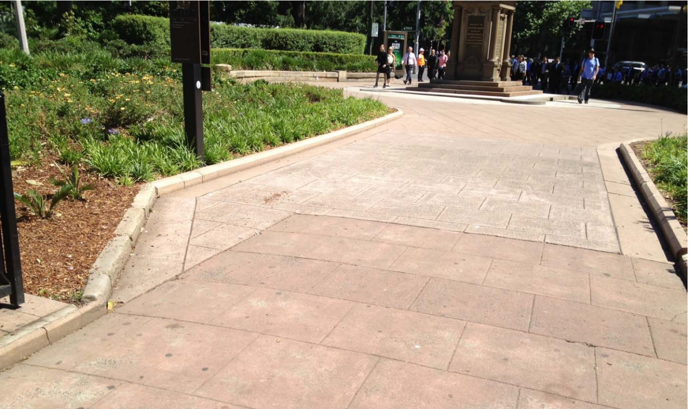
Image c) Inconsistent use of pavement materials
